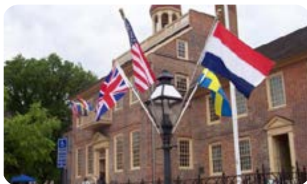
New Castle Courthouse
